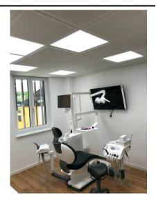
Dentled panels are available in the standard suspended ceiling measurements of 595×595, 625x625(Germany) and 1200×300. Next to treatment rooms Dentled panels are often applied to hallways and dental sterilisation rooms to ensure an optimal light transition from the personnel routes to the rest of the practice. For sterile rooms Dentled fitted panels are preferable to suspended fixtures for reasons of hygiene.
